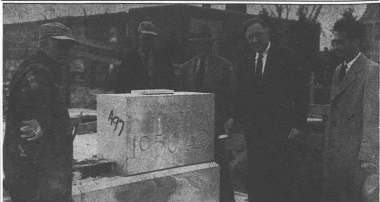
At a brief ceremony held last Wednesday in front of the Delsell Hall construction, the cornerstone for the men's dorm was laid, with President William C. Hansen doing the mason work. Dr. Warren E. Jenkins delivered a short address at the ceremony. Pictured above (l. to r.) Harry Weedman, Stevens Point, Emil Jorgensen, building superintendent of Oshkosh, Elliot Kaiser, state building superintendent of Madison, President Hansen and Dr. Jenkins.
