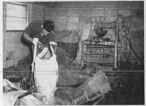
Construction continues towards the completion of the third floor of Delzell Hall. Until third floor is completed, the residents are being housed elsewhere.
