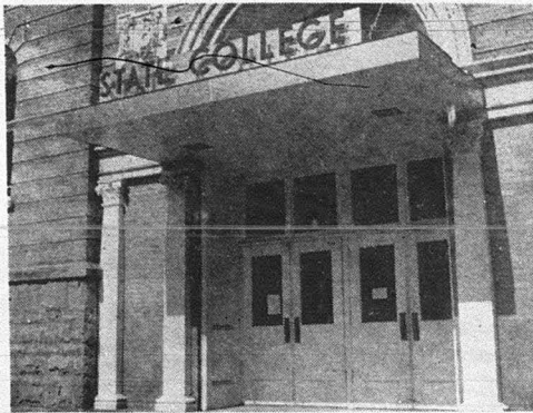
Improvements were external as well as internal here at CSC as this picture of the new sign over the main entrance shows.
