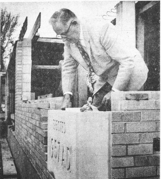
President William C. Hansen is shown here as he places a copper box containing newspapers and other documents inside the corner stone of the new CSC dormitory. (E. Specht photo).
