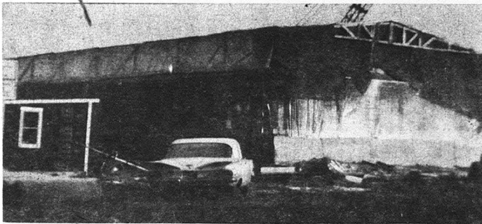
WINTER CONSTRUCTION of new CSC dormitory.
