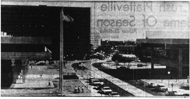
THREE OF THE EAST-WEST CENTER'S complex of six buildings designed by architect I. M. Pei of New York are, from left, Thomas Jefferson Hall, the
