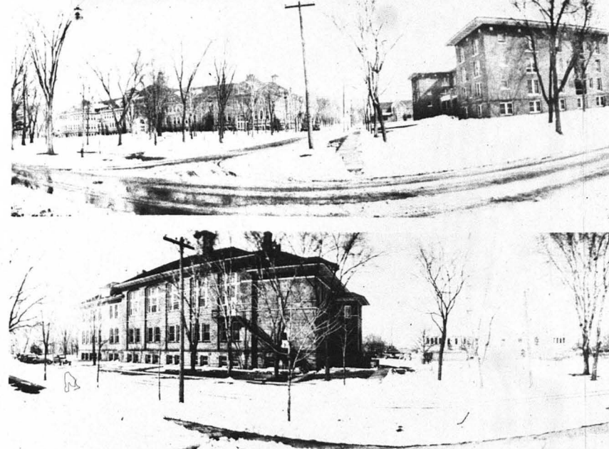
THE TOP PICTURE shows Old Main in a winter setting from across Main Street directly in front of Old Main. The bottom photo shows the construction of what today is called the Campus Lab School. The top photo was taken in 1929 while the bottom in 1927.
