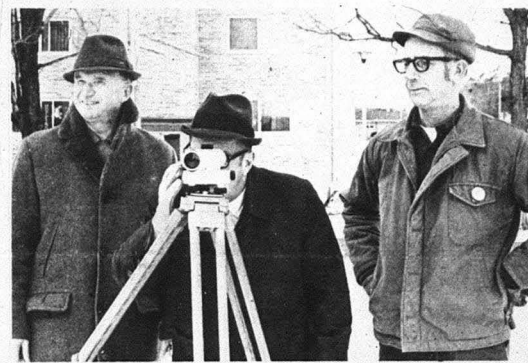
WITHOUT THE FANFARE of groundbreaking ceremonies, construction got underway on a new $190,000 building at Stevens Point State University to house a Centrex phone system and the offices of security and protection and director of the physical plant. From left are Nels Anderson of Ellis Stone Co., Stevens Point; Hiram Krebs, director of the university physical plant; and Charles Sharp, Edgar, superintendent for Ellis Stone. Meanwhile groundbreaking program was taking place on another part of campus for a new $2.4 million classroom building.
