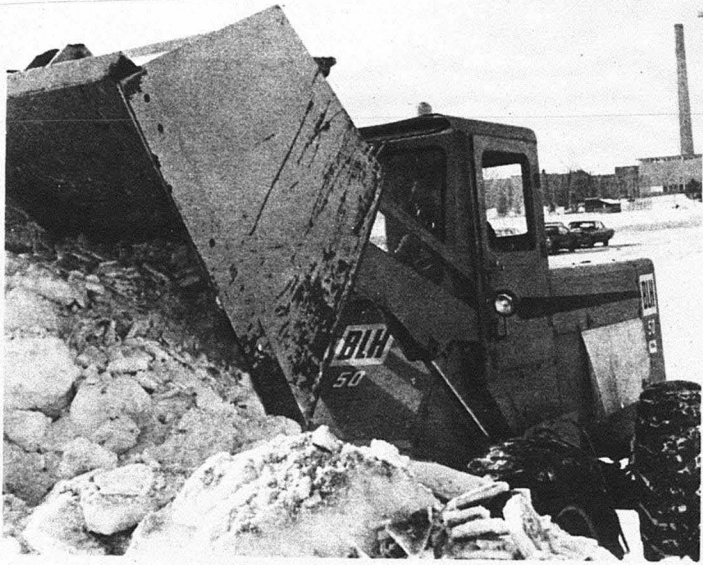
Snow removal requires hard work and many long hours.
