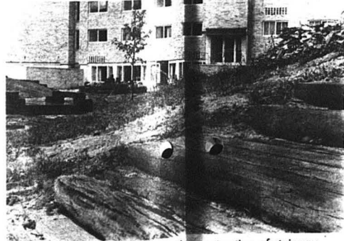
Old railroad ties were used for construction of stairway (foreground) and wooden bridge (center left)
