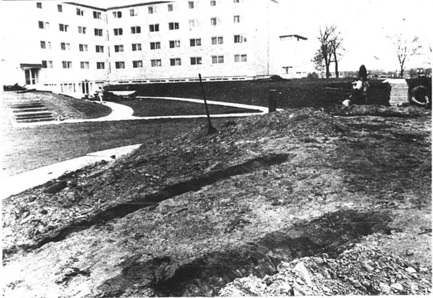
In the beginning there was only mud and trenches.
