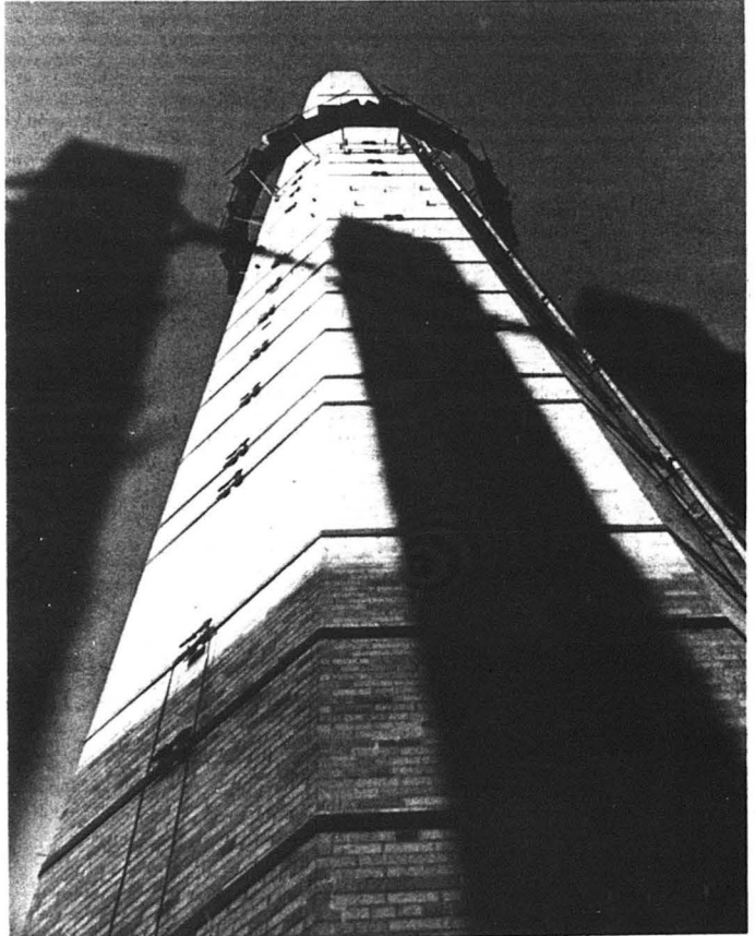
A worm's eye view of repair work being done on the smokestack. Photo by Bill Paulson.
