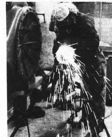
Welder works on UWSP's $565,000 energy modification project in Collins Classroom Center. Recently, the project was tabbed "a disaster" by UWSP Administrator Zeke Torzewski. (Photo by Rick McNitt)
