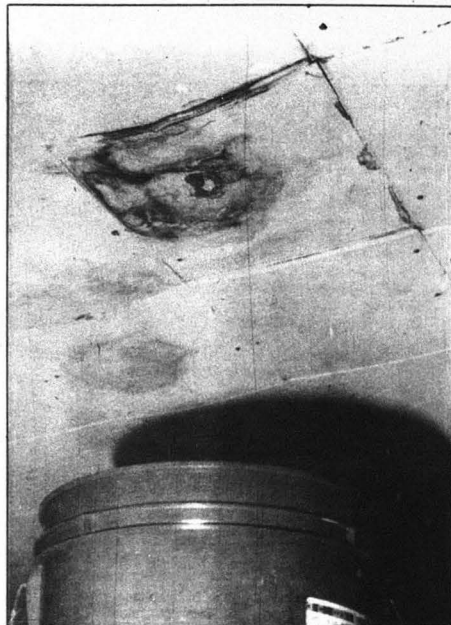
Dan Smith's "own waterfall" and the bucket which is used to catch water which leaks from the first floor bathroom.
