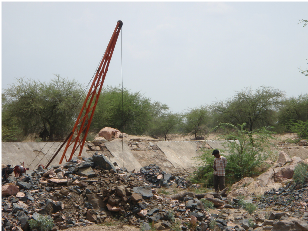
Figure 8. Well under construction near Sanjadi-ka-badia, India. Photo/Lindsey Wood.
