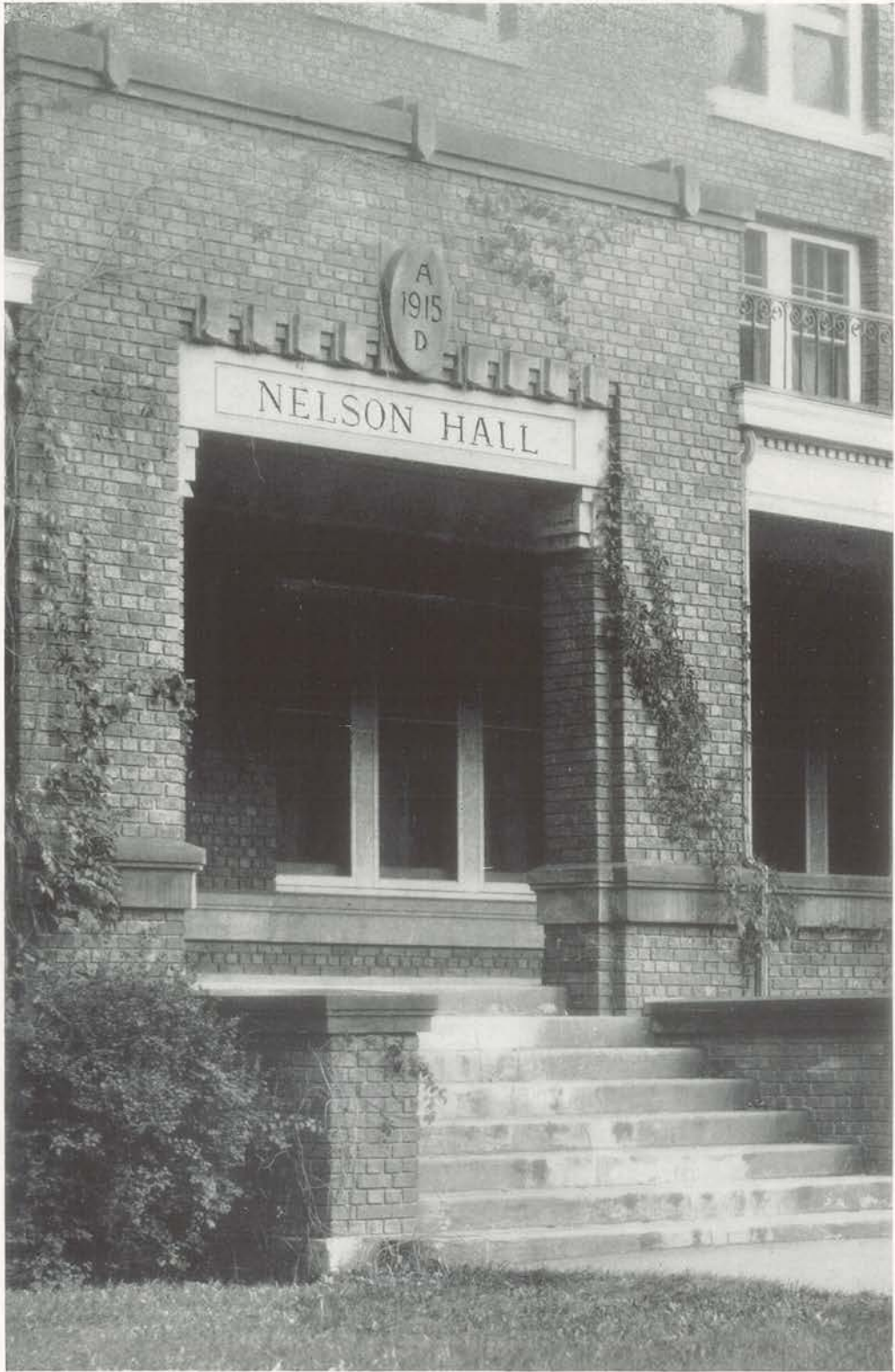
NELSON HALL ENTRANCE
