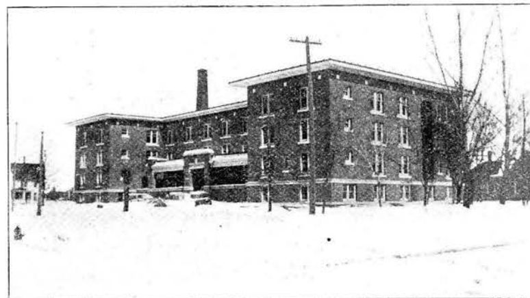
NELSON HALL, EXTERIOR VIEW
