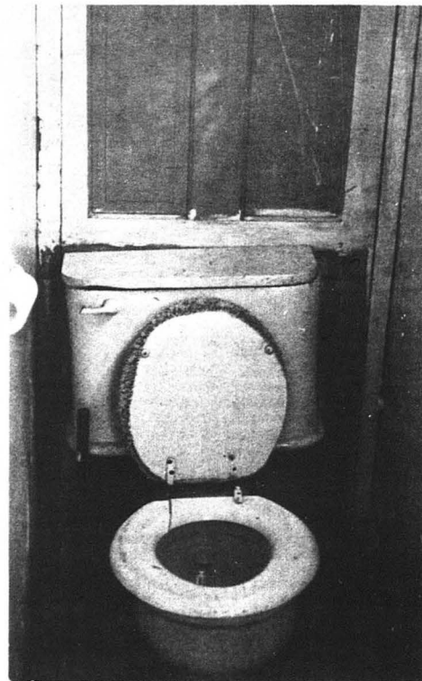
This is the entire bathroom complete with no dor. A shower is located on the other side of the apartment.
