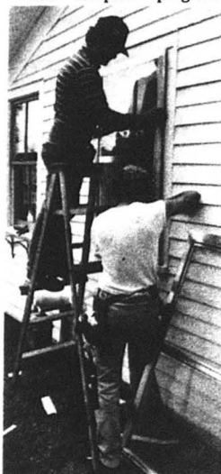
CAP workers install storm windows
