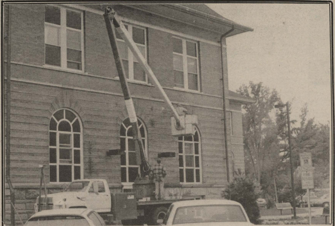
Old Main not only gets cleaned inside, but outside too throughout this week. (photo by Jeff Kleman)
