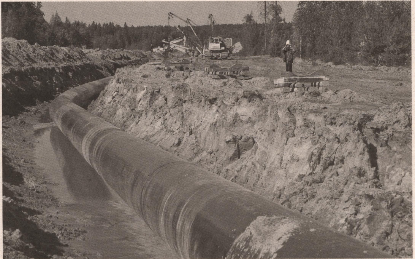
Construction of a pipeline. Photo courtesy of NPCA Online
