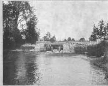
Paper Mill Bridge
